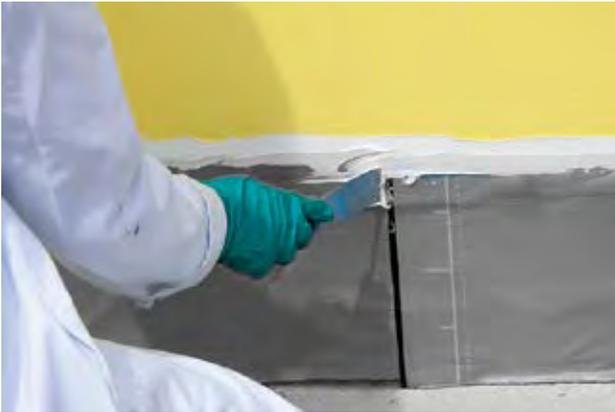
Example of bridging from below grade water proofing to Air Barrier using *Dow Corning*<sup>®</sup> 758 Silicone Weather Barrier Sealant
