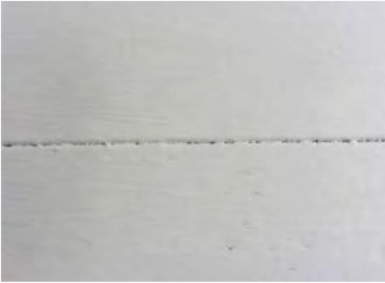
**Post application inspection shows sheathing joint not properly sealed. Reseal with sealant.**
