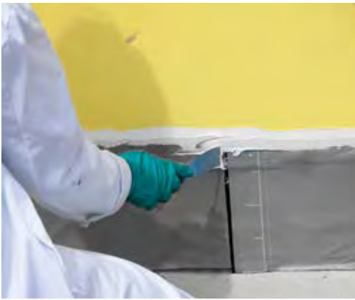
Example of bridging from below grade water proofing to Air Barrier using Dow Corning ® 758 Silicone Weather Barrier Sealant
