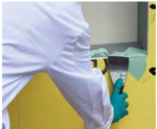
Example of using Dow Corning® 778 Silicone Liquid Flashing
