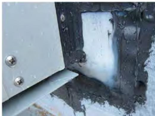
Figure 4: Sealant Attaching Strip and Corner to Air Barrier In-field. Lap Joints Sealed.
