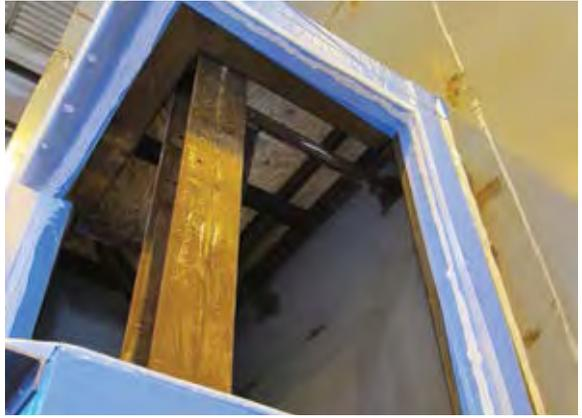
**Figure 7: *Dow Corning*<sup>®</sup> Silicone Transition System-Wrapped Opening**
