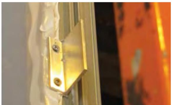
**Figure 10: Mechanical Fasteners May Be Used with *Dow Corning*<sup>®</sup> Silicone Transition System. (Sealant Also Must Be Applied Over This Fastener and Tooled.)**
