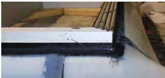
Figure 2: Corner and Strip Pieces Installed In-shop
