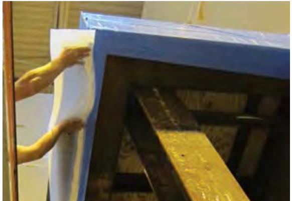
**Figure 9: Installing Strip at Head of Fenestration Unit Using Sealant**
